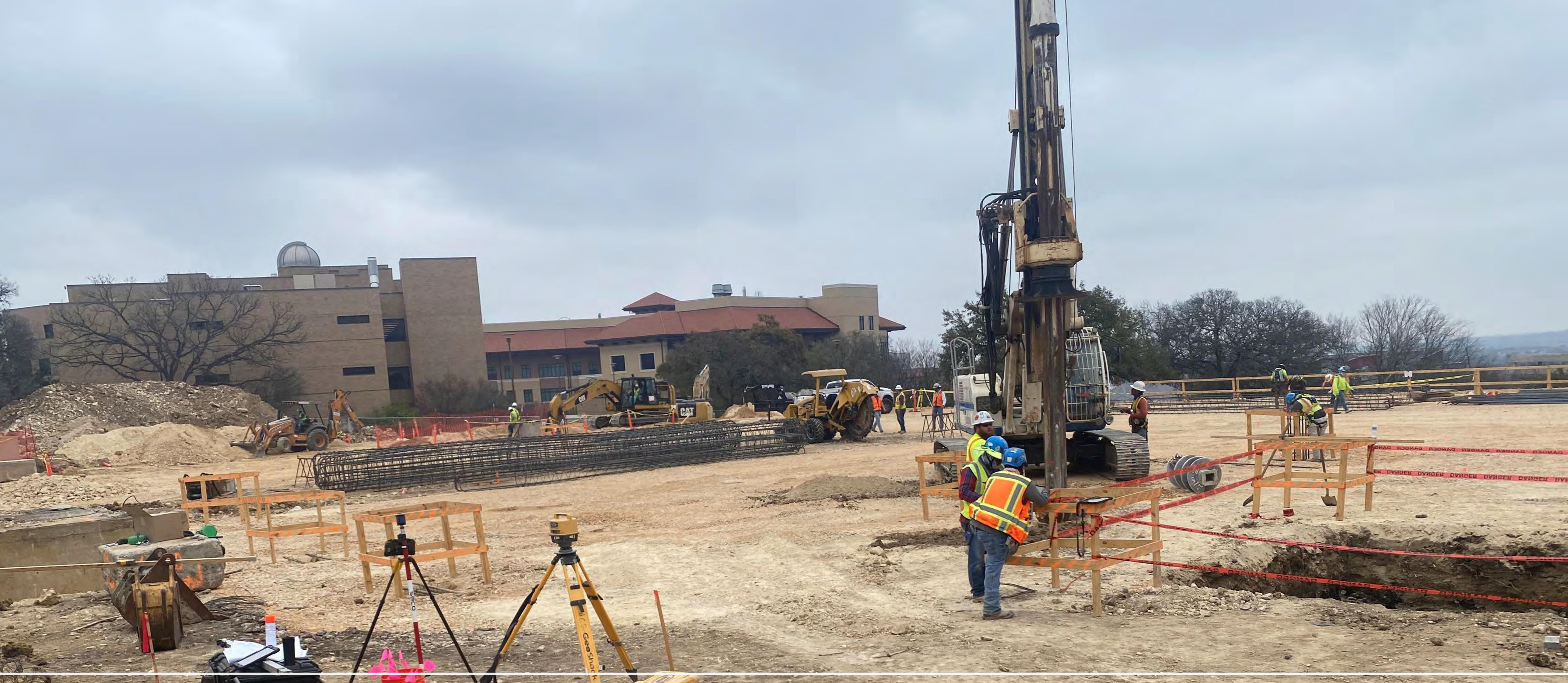
Canyon Residence Hall- Bldg. Pad
